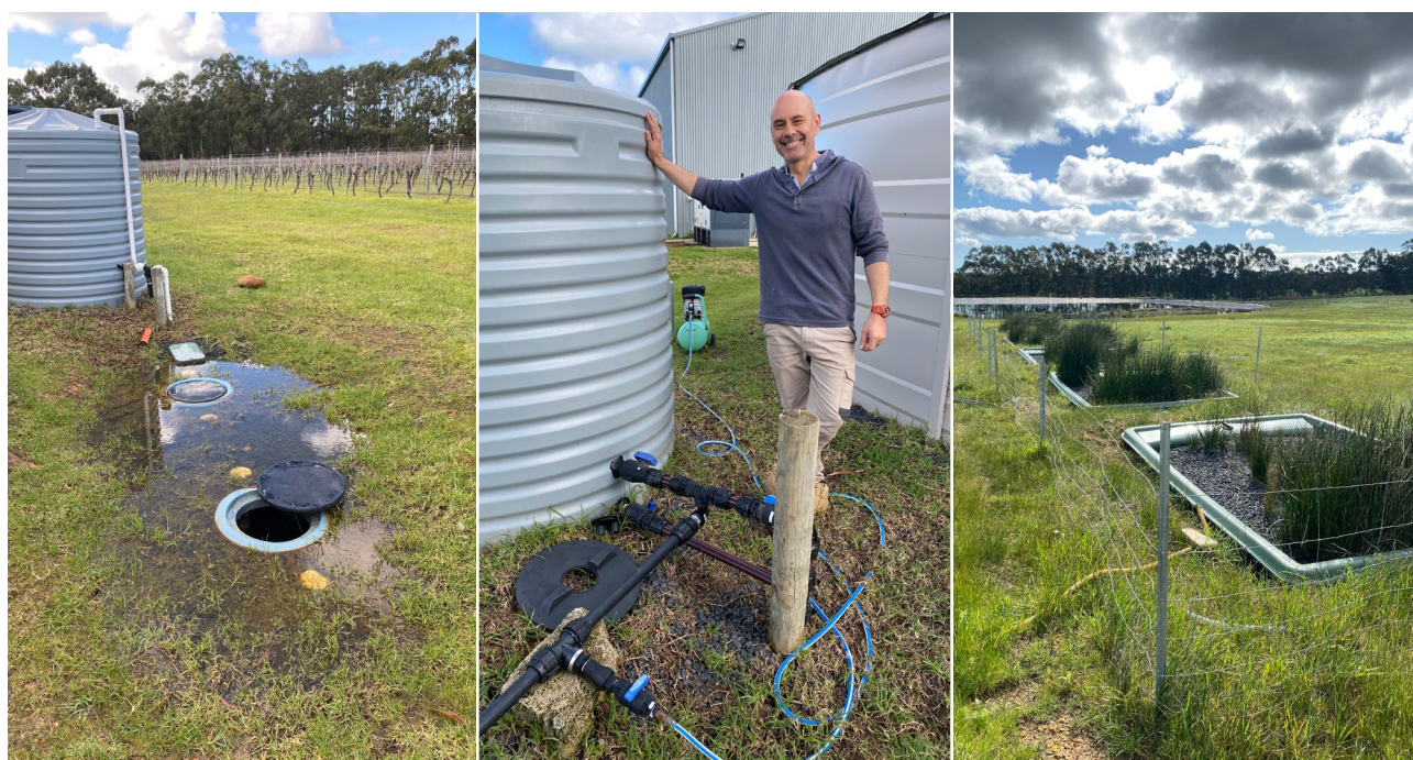
Figure 6. Baffle tanks are in the foreground (left), with wastewater pumped to the treatment tank that can be circulated for aeration and pH adjustment (centre) before being stored in the 22 kL tank (not pictured) and sent to the five reed bed pods located downhill, halfway between the winery and dam (right). Images were taken in August 2022 following significant rain, water visible around the baffle tanks is ground water.
