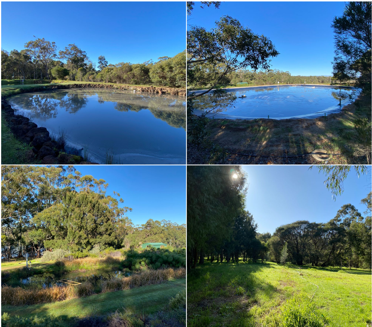
Figure 3. Ground level view of the two treatment ponds (top left two anaerobic ponds, top right aeration pond), papyrus reed beds (bottom left) and irrigation woodlot (bottom right). The woodlot shows mature eastern river sheoaks (22 years old) and recently planted saplings. Irrigation lines can be moved throughout the woodlot.
